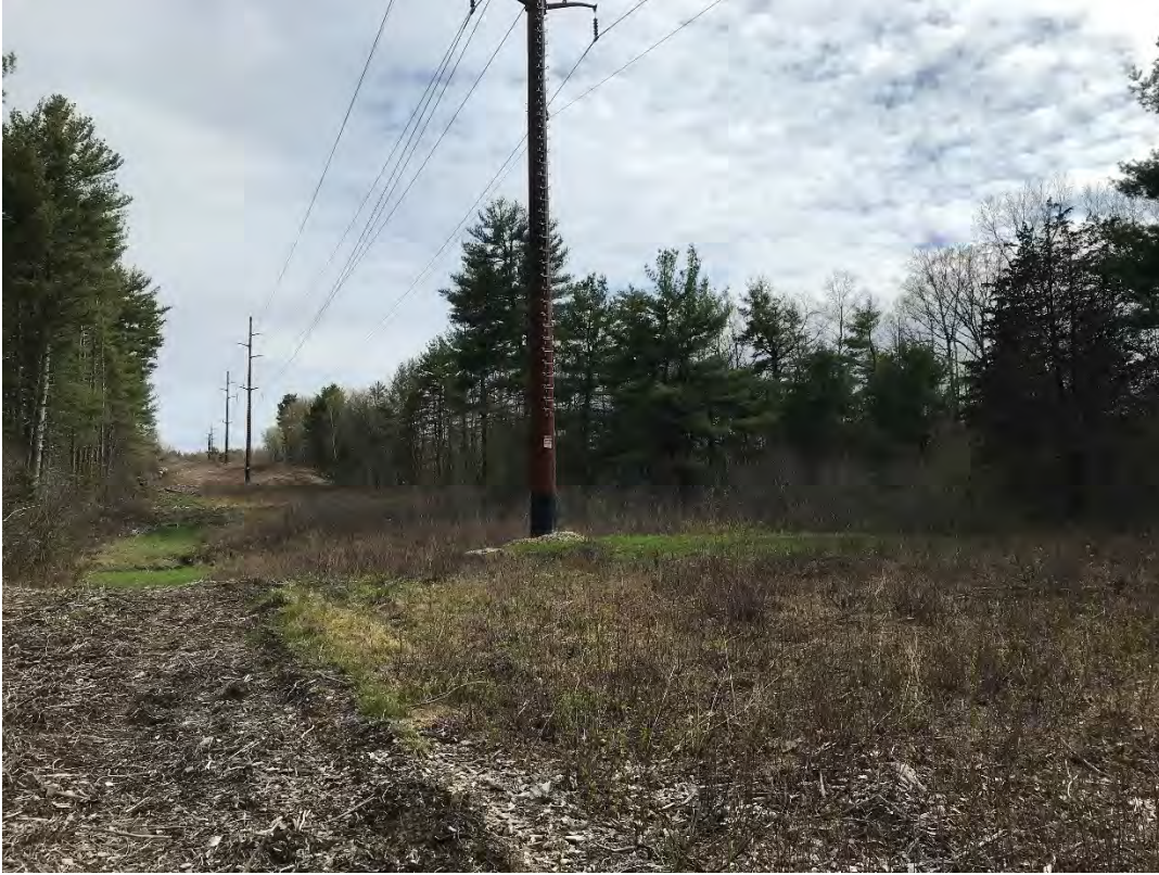
Fig 13: Str. 44 work area with adjacent access route and stream DS60. Viewing south. (05-04-21)
