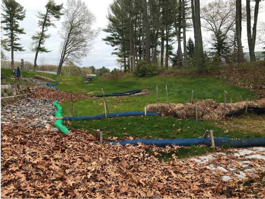
Fig 9: Slope above the manhole at Gundalow Landing/east side of the bay. Viewing east. (05-04-21)
