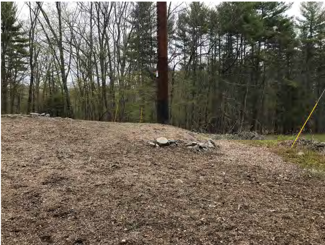
Fig 6: Str. 90 work area. Viewing northeast. (05-04-21)
