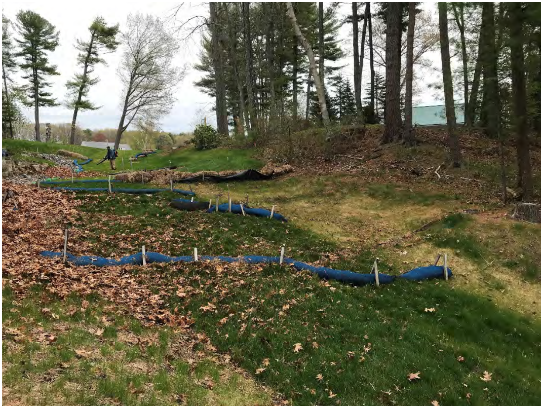
Fig 10: Slope below the manhole at Gundalow Landing/east side of the bay. Viewing east. (05-04-21)
