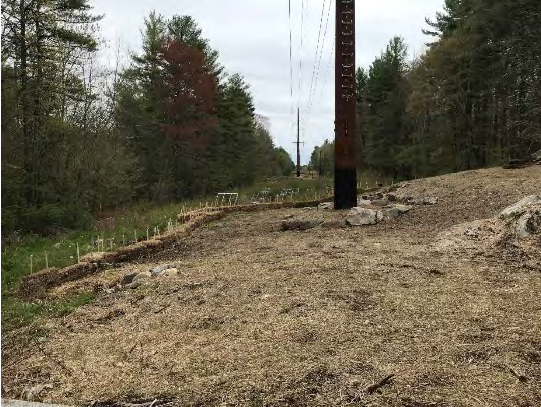
Fig 5: Str. 89 work area. Viewing southeast. (05-04-21)
